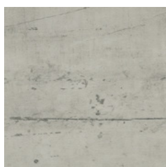
p40 Cold Cracked Concrete
