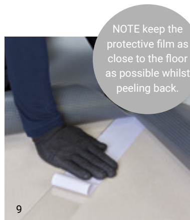
9 Carefully peel away the protective film from all areas where the tape has been applied.
